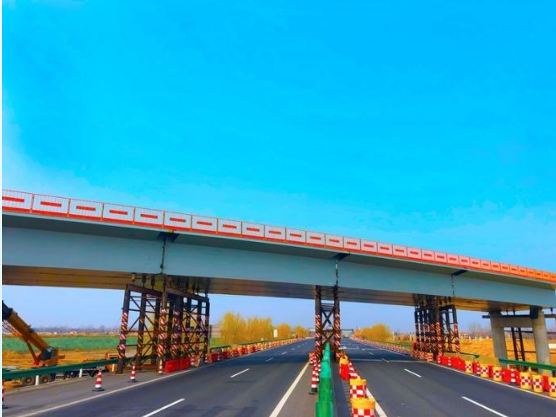
Automotive bridge metal structure
